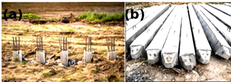
Plate (1) concrete piles
